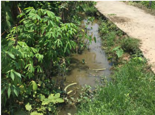
Photo 7: A section in Loi Ma – Cau Ngao drainage canal
