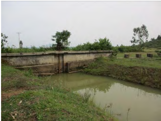
Photo 1: The existing spillway of Lower Khe Hao Reservoir
