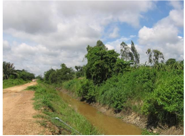
Photo 2 Status of North Ba Bau main canal to be upgraded
