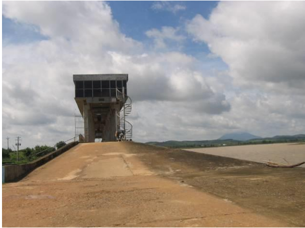
Photo 1: Ba Bau Dam & Reservoir
