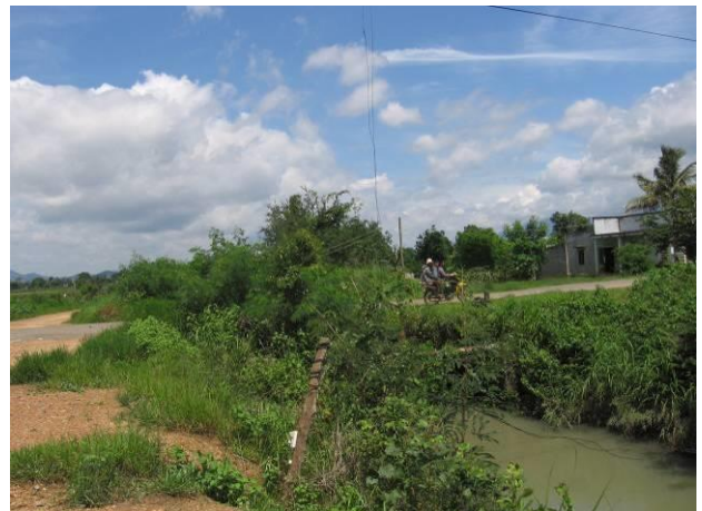
Photo 4: Intersection point of Province Road No 707 & upgraded Bac Ba Bau main canal; Air quality monitoring & water quality & Public Safety monitoring point
