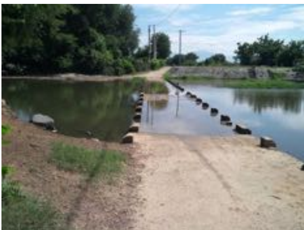
Photo 5. Overflow location on the main Southern canal, intersection point with Lanh Ra
