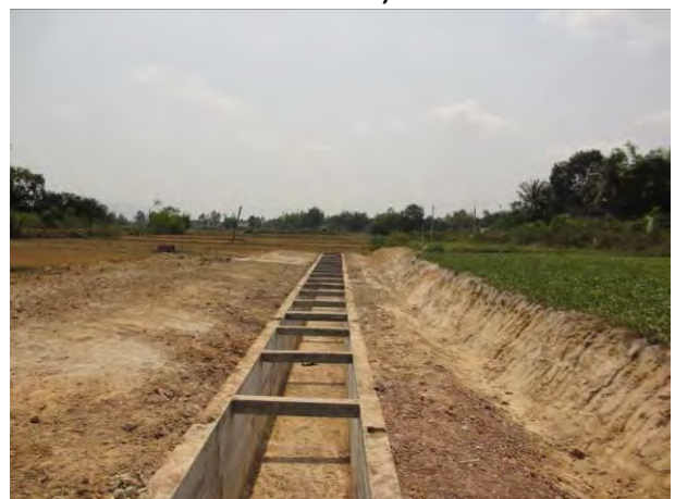
Photo 14: The end of existing main canal N24, Thuan Hanh hamlet, Binh Thuan commune
