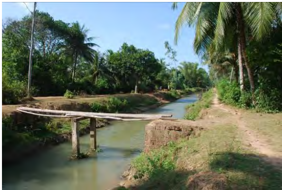
Photo 1: Main canal in Hoai Hao Commune
