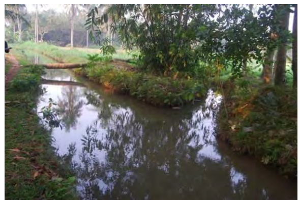
Photo 4: N2A Canal in Hoai Xuan Commune
