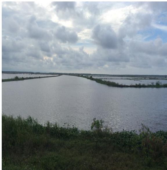
Easten side of Hoi Tom protection Dike
