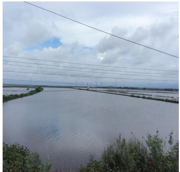
Westen side of Hoi Tom protection Dike
