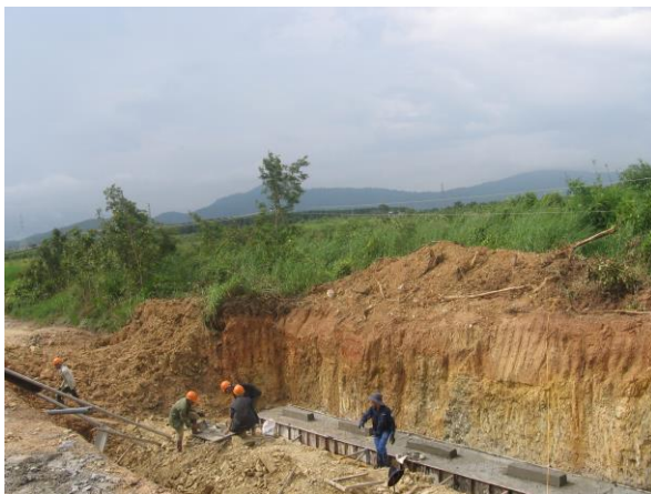
Main canal –Lot 2 of Ba Bau Subproject
