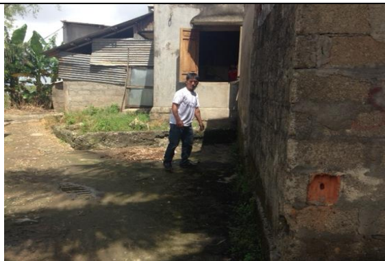
Affected temporary house in Loc An commune
