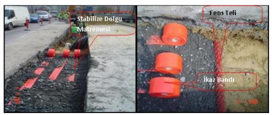
Figure 20. Warning band, fence wire and stabilized materials
