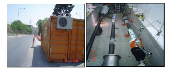
Figure 21 Underground Cable Splicing Points
