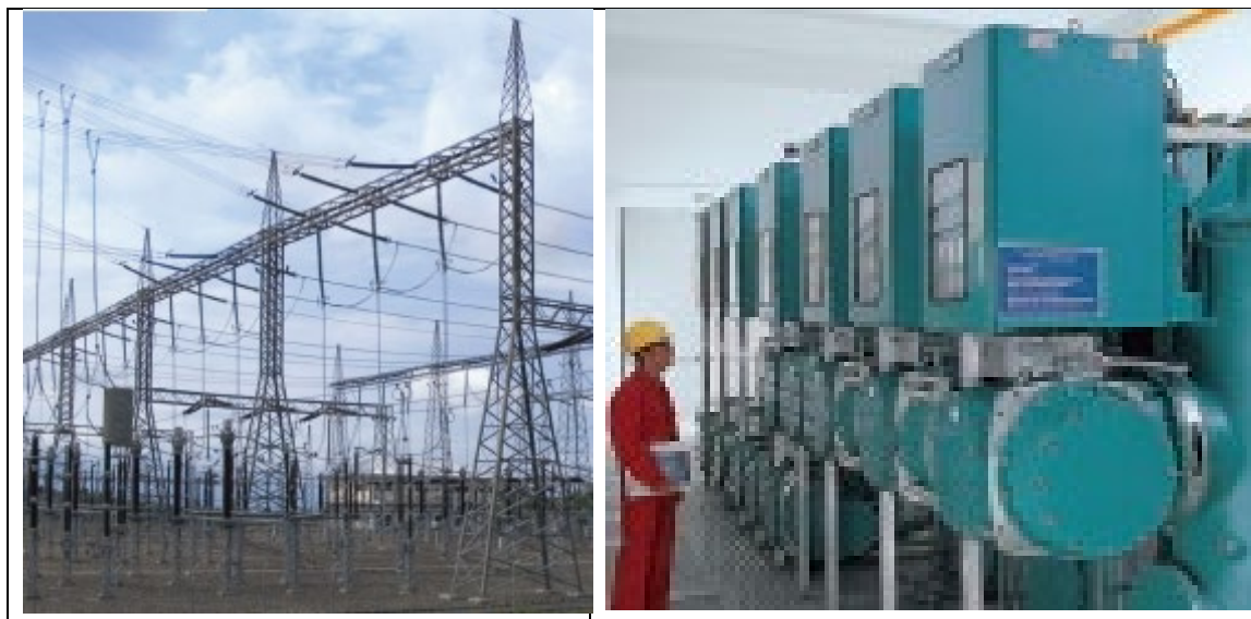
Figure 3-8: AIS (left) vs GIS (right) substation
