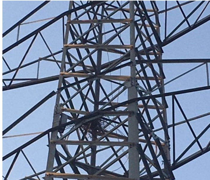
Figure 7-1: Nests in Towers 220 kV TL from Rawat to University Grid (Ankara Park Islamabad)
