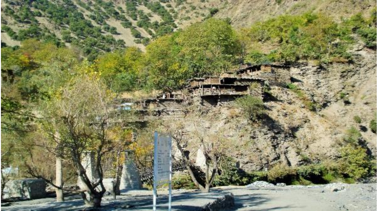
Picture-14: Typical wooden housing structure in Kalasha valley
