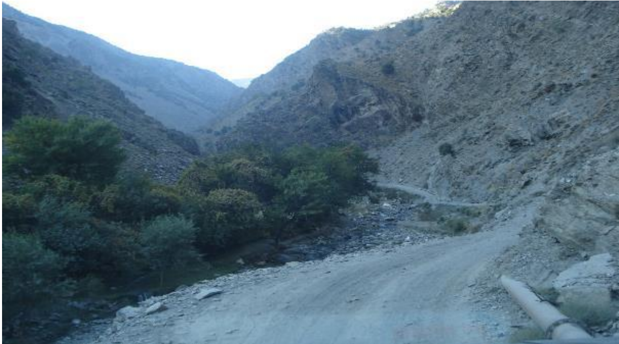
Picture-12: Road condition from Birir to Chitral
