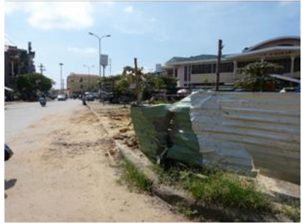
Safety fences for PS construction sites
