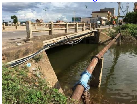
Existing pipes parallel with the bridge
