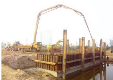
Construction of bridge piers
