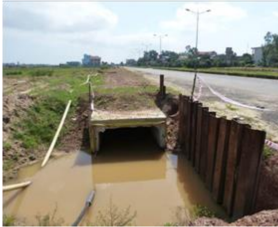
Larsen sheet piles are deployed to prevent land slump during drain construction
