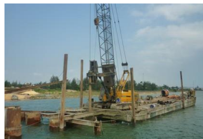
Construction of bridge abutments
