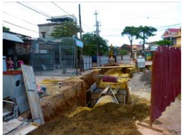
Safety fences during road excavation for pipe laying
