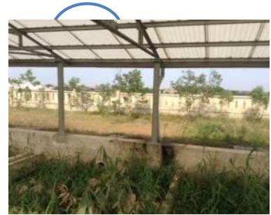
Sludge storage area with roof, surrounding wall and grass to mitigate pollution
