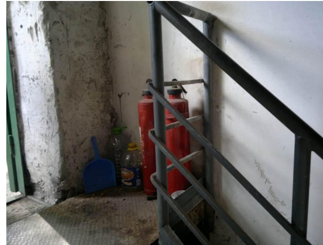
Picture 2. GHS in Chisinau, fire extinguishers
