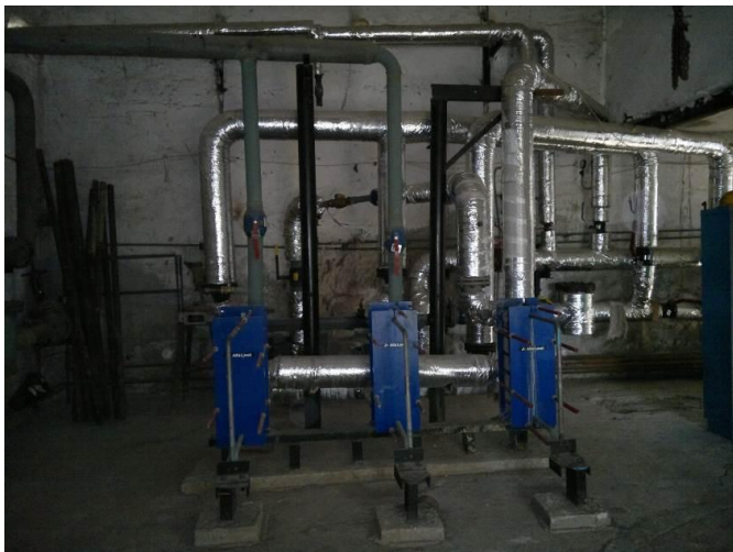
Picture 3. GHS in Chisinau, heat exchangers
