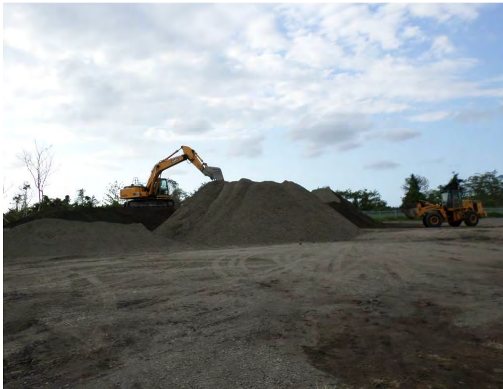
Picture 13: Proper stockpiling away from water bodies and secured clean working area
