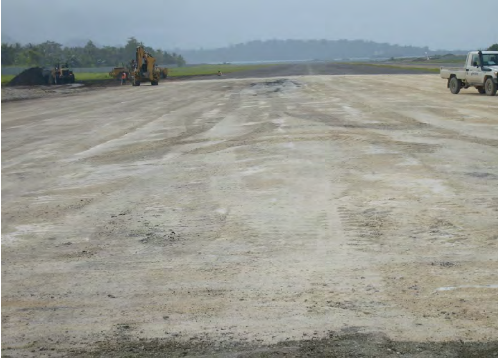
Picture 14: Grubbing and scrubbing; topsoiling and proper stockpiling begins. Water truck is issued to control dust.
