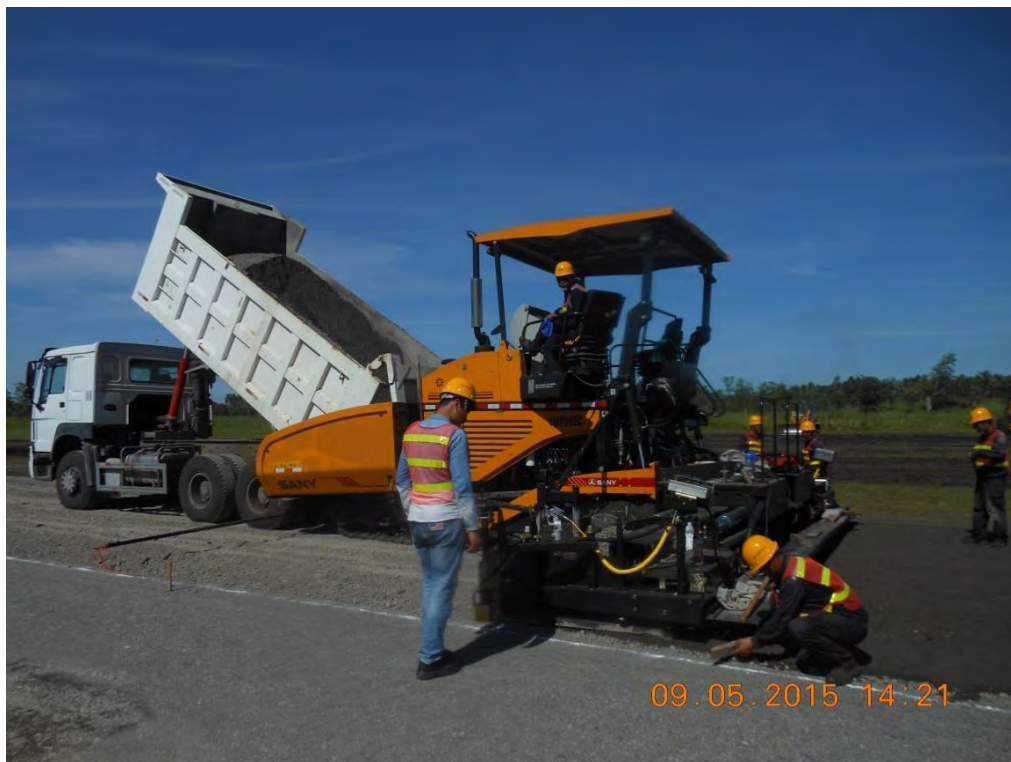
Picture 4: Laying of the basecourse materials on the new design level at the main runway. Notice moisture content of the basecourse to control excessive dust emission.
