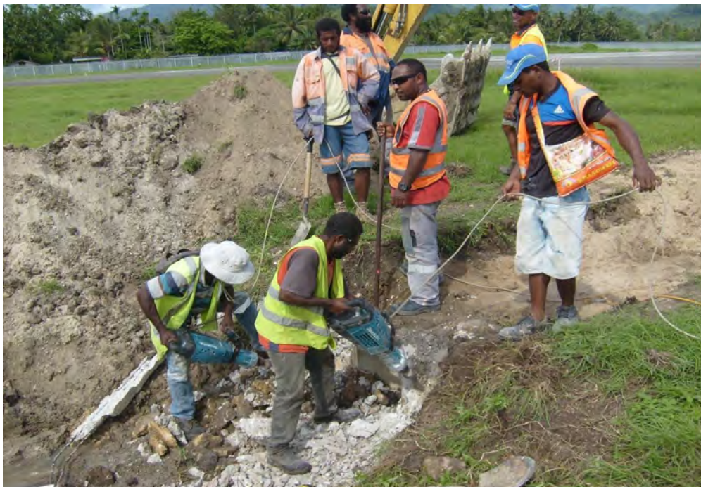
Picture 15: Clearing and trenching for the 6m fence-line corridor for new palisade fencing installation.
