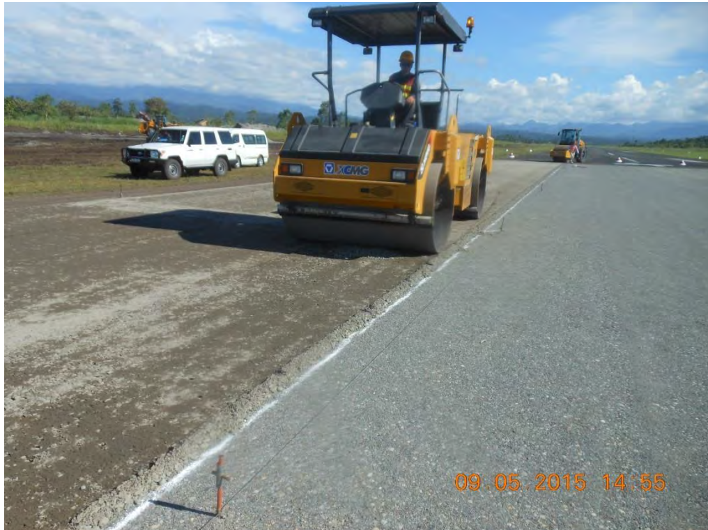
Picture 3: Compaction of the basecourse materials on main runway. Notice moisture content of the basecourse to control excessive dust emission.
