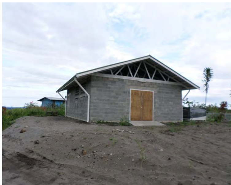
Picture 10: Completed new stand-by generator shed. Notice that it is housed-in as a buffer to control noise pollution
