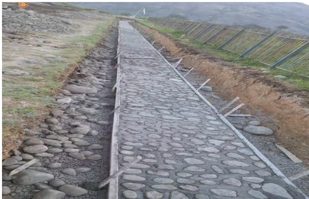
Picture 20: Construction of line drain close to the fence-line commence soon after excavation. High rainfall pattern including the exposed soil can easily be washed off if exposed so it is concreted to minimize sedimentation.
