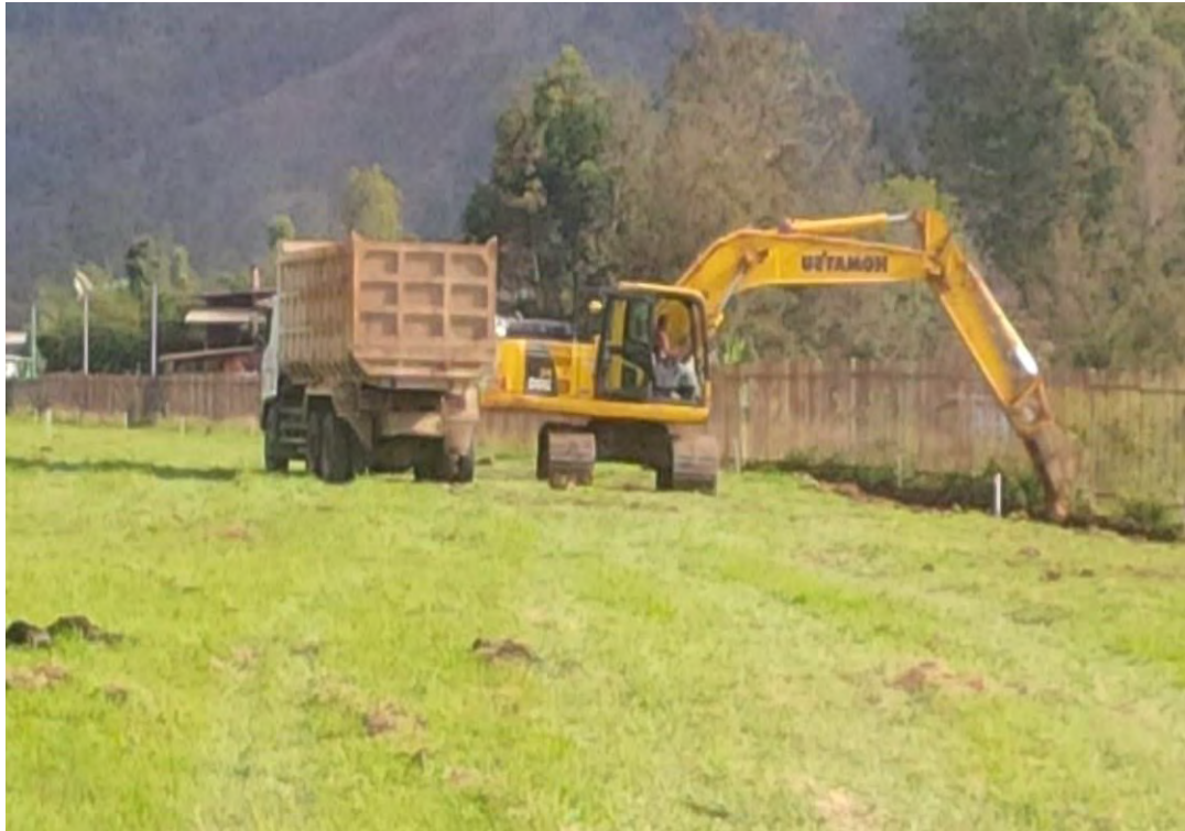
Picture 19: Grubbing and scrubbing; topsoiling and excavation begins for the construction of lined drain.
