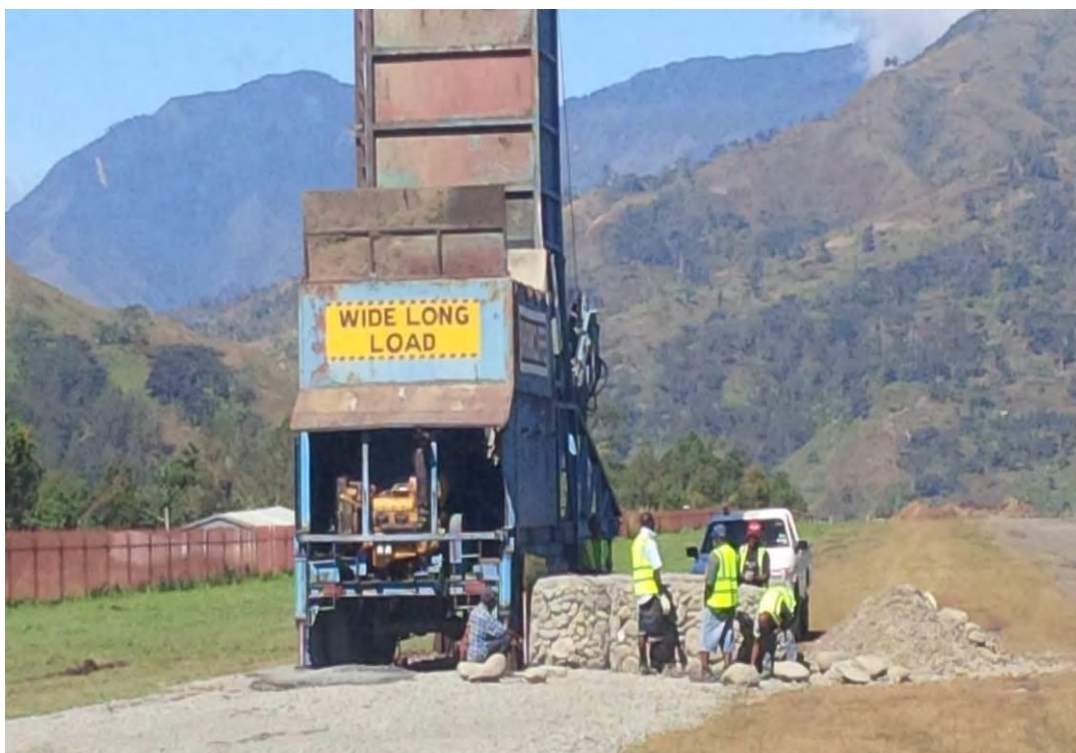
Picture 21: Assembling of the crusher parts inside the airport. Preparing and stabilizing the area for aggregates stockpiling next to the crusher.
