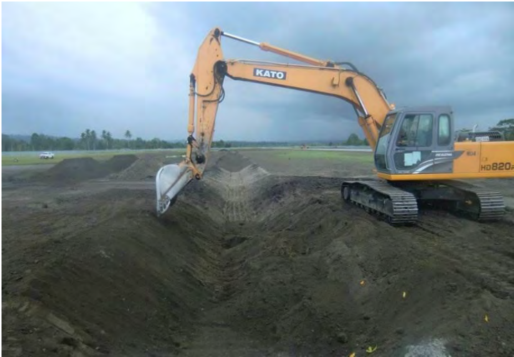
Picture 1: Grubbing scrubbing; topsoiling and proper stockpiling. Constructing of open unlined drain (OUD) with proper dimension design to collect and drain off surface runoffs at the highest rainfall.
