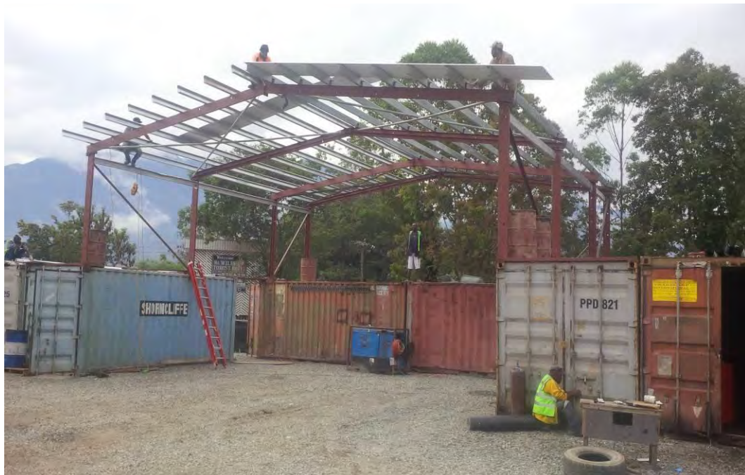
Picture 18: Construction of the contractors' workshop. Containers will be used as the storage rooms for vehicles/machineries parts and petrochemical products. Any spillage will be contained inside the container and cleaned immediately without being exposed to the soil.
