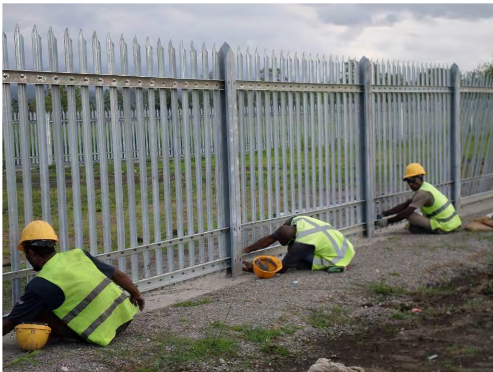
Picture 5: Installation of palisade fencing works done by locals.
