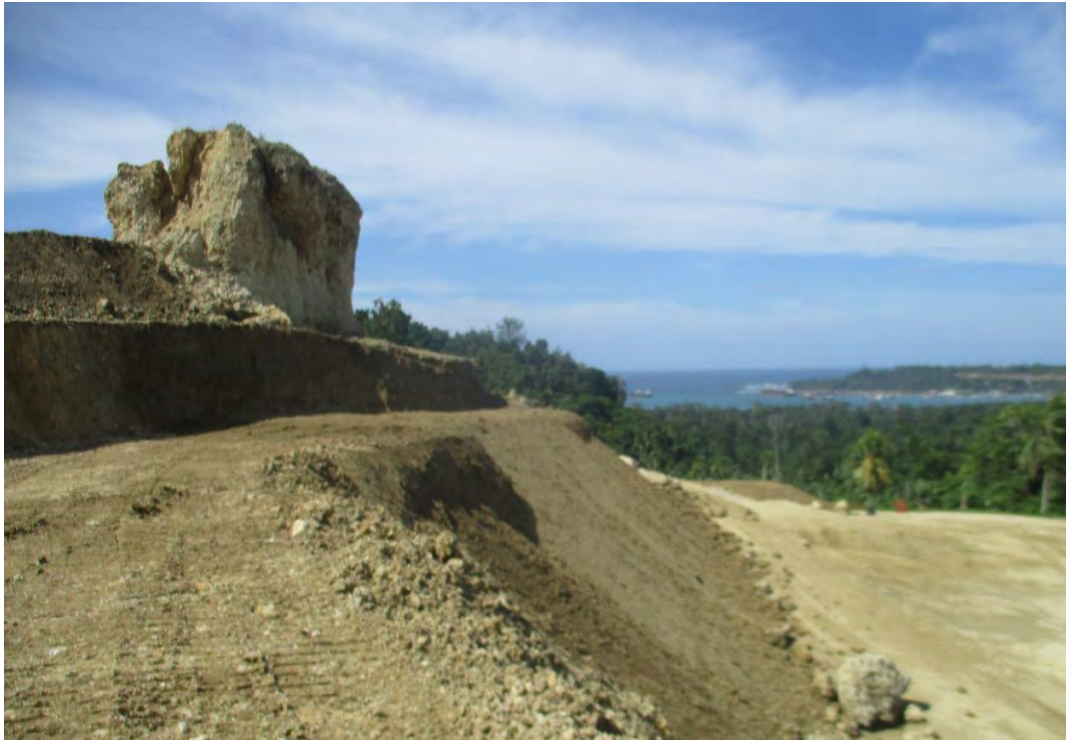
Picture 16: Extraction of base course and sub-base is taken from coronus materials. The site is disturbed and away from local communities and surroundings.
