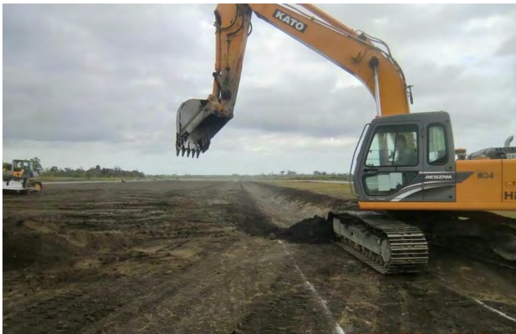
Picture 2: Works undertaken at the designed alignment of the open unlined drain (OUD). Earthworks stockpile is immediately disposed at stockpile area away from the drain and later used for topsoiling and re-grassing
