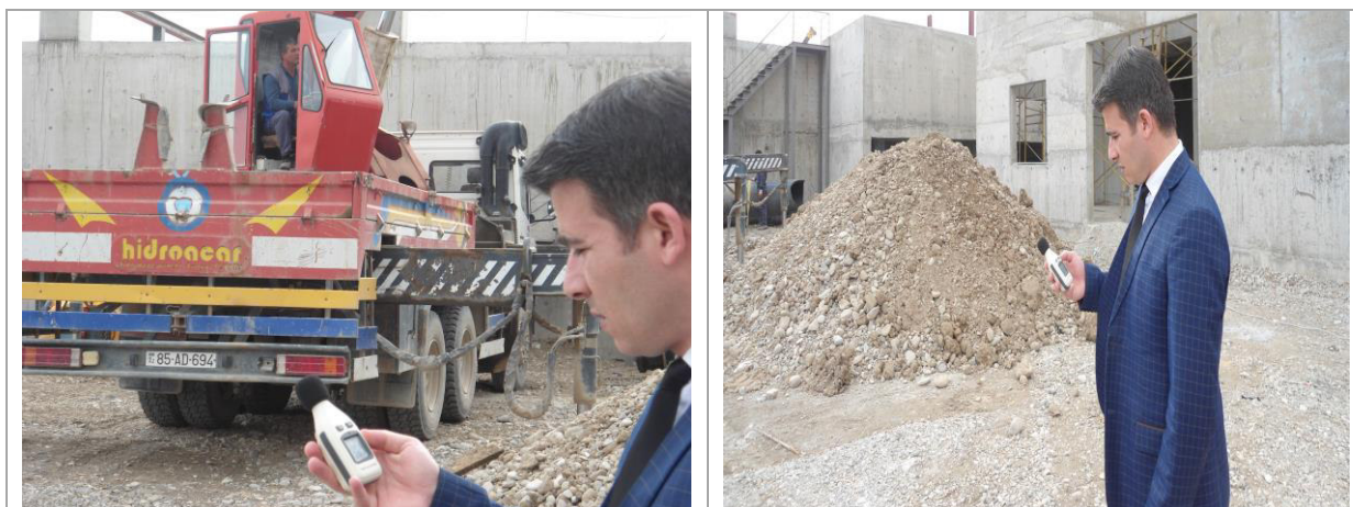
Figure 3: Noise and Dust Measurement Equipment at Project site
