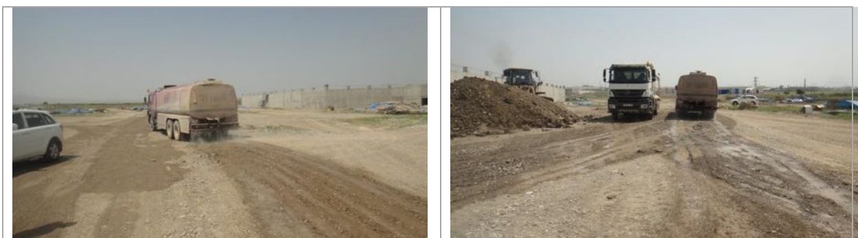
Figure 2: Dust Control at Project site
