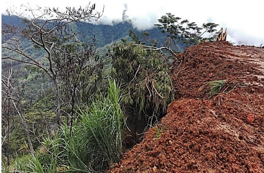
Photo 6 Damage to Natural Vegetation resulting from road spoil dumping
