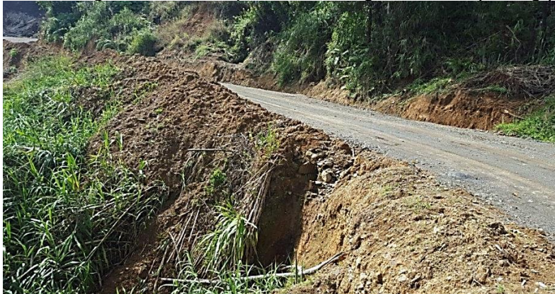
Photo 3 Construction Spoil Rolled Down from slopes above
