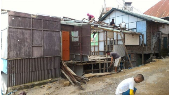
Mr. F. Lalengliana's, Zotlang, House during dismantling
