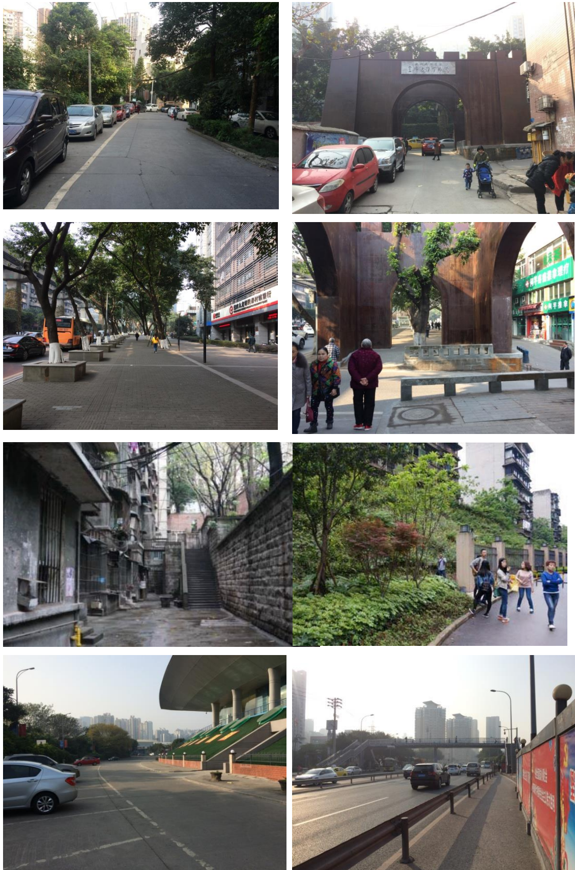
Figure 3.2-5 The status of the footpath phase III project
