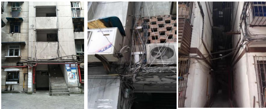
Figure 4-5 Disorderly wiring
