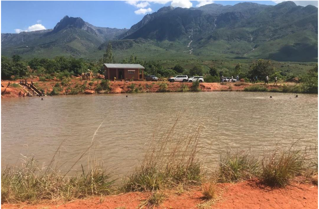
Figure 2.6: Existing Night Storage Reservoir
