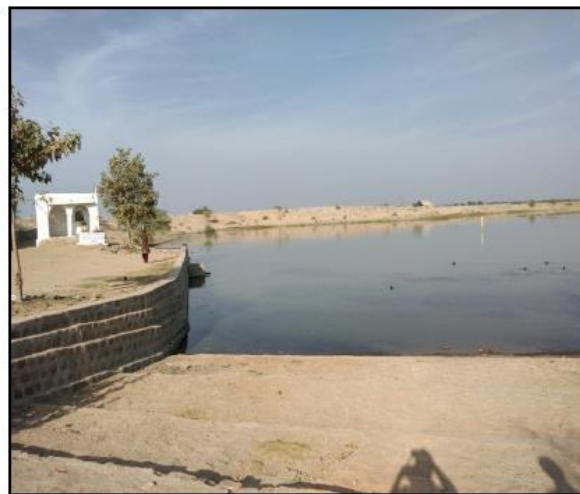
Pond at Asop at 78+650 on RHS
