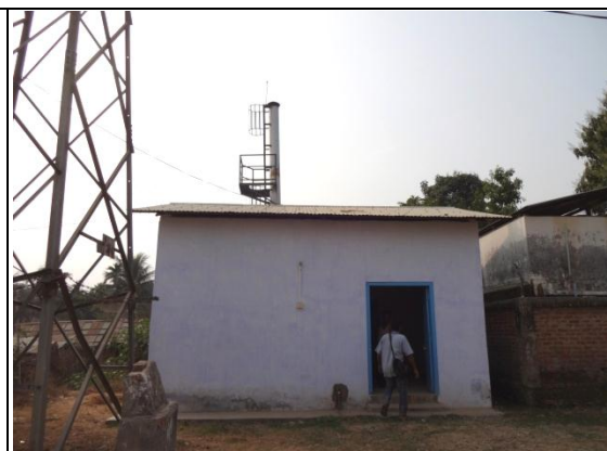
Incinerator at Dimapur District Hospital
