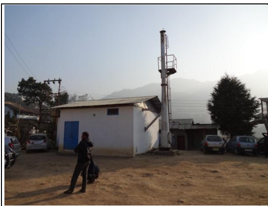
Non-functional Incinerator at Naga Hospital at Kohima
