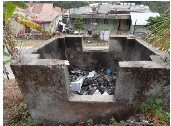
Burning pit used in Viswema CHC for all waste including bio-medical waste
