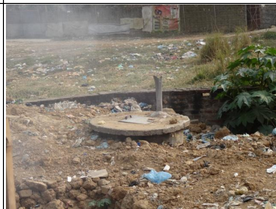
Pit for sharps at Dimapur Dist. Hospital
