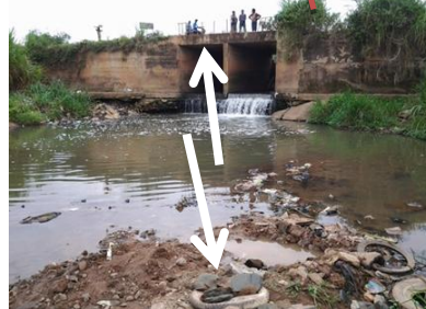
Plate 5: Dilapidated bridge and heavy siltation
