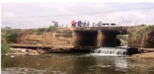
Inadequate culvert with collapsed walls; lack of protective barriers Road undercutting; Land degradation
