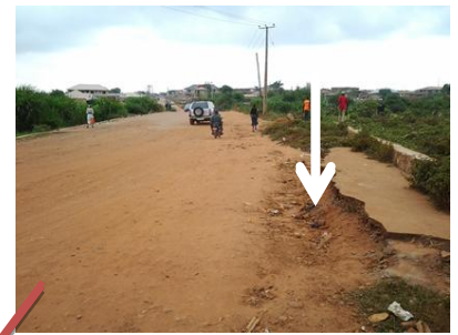
Plate 3: No drainage on approach roads
