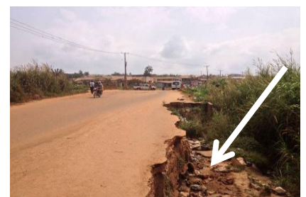
Plate 9: Road undercutting;
