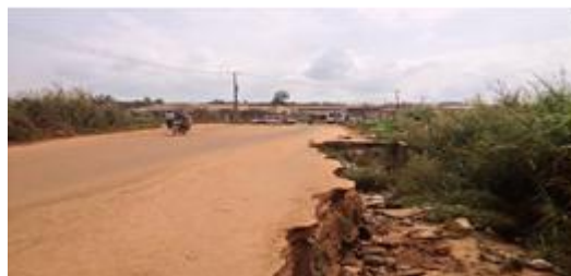
Inadequate culvert with collapsed walls; lack of protective barriers Road undercutting; Land degradation
