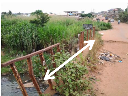
Plate 7: Damaged Cross Bar
