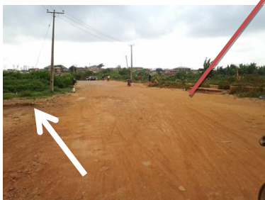
Plate 4: No drainage on approach roads
