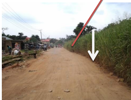
Plate 4: No side drains on approach road
