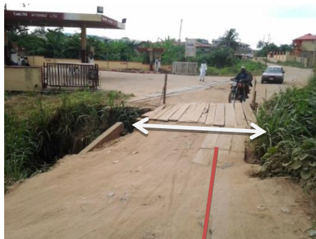
Plate 2: Narrow width of existing damaged culvert
