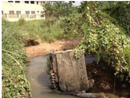
Collapsed culvert in downstream
