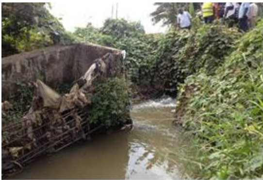
Collapsed culvert on the river bed
