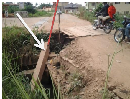
Plate 5: Existing damaged culvert structure
