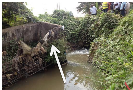
Plate 1: Collapsed culvert on the river bed
