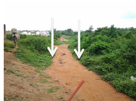
Plate 3: No side drains on approach roads
