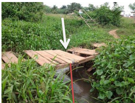
Plate 2: Dilapidated make shift cross over
