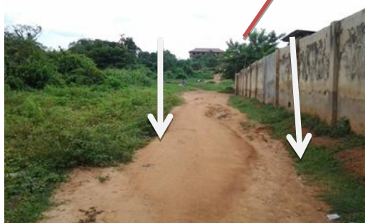
Plate 5: No side drains on approach roads
