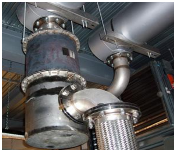
Exhaust systems incorporating diesel particulate filters
