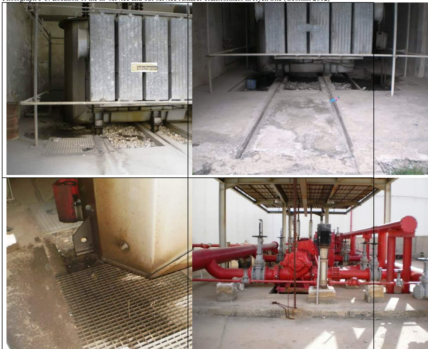
Photograph 5-6: Oil Leakages from the in-service Askarel Transformers in Jiyeh Site (Geoflint 2012).
