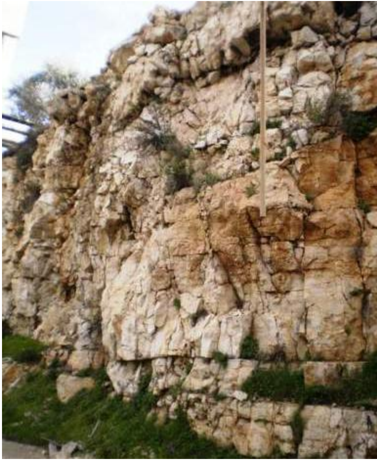
Photograph 5-8: Exposed geological formation at Jiyeh site (Geoflint 2012).
