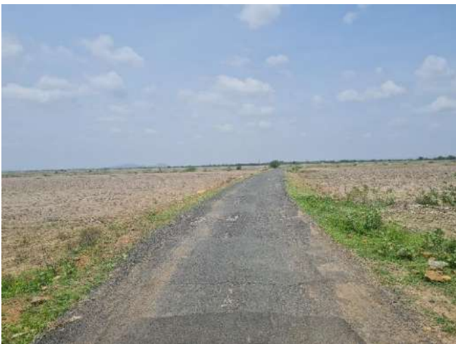
Access road to site
