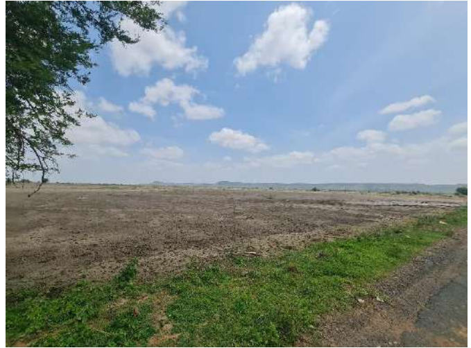
Solar Plant Site
