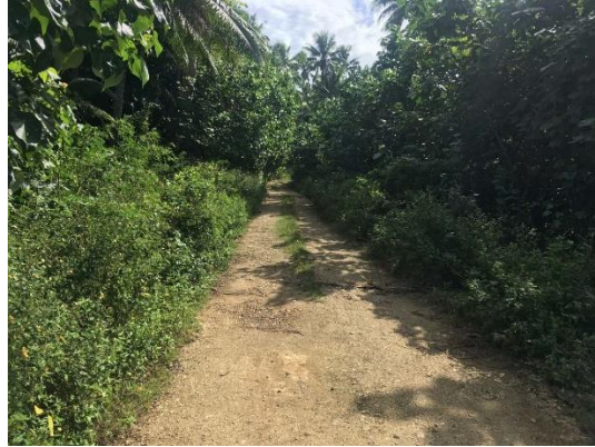
Rural road, Pangai, Lifuka, Ha'apai
