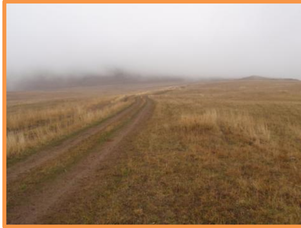
Figure 1-3. Existing Rural Road 4km from M2
