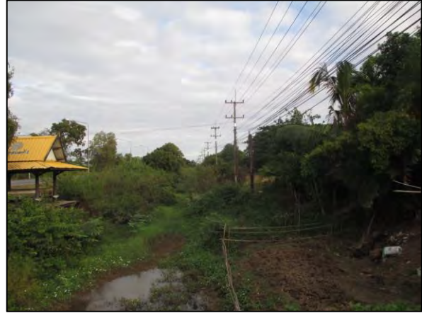
Open side drain in Phan Na Village is clogged with vegetation and reportedly swell during heavy rains
