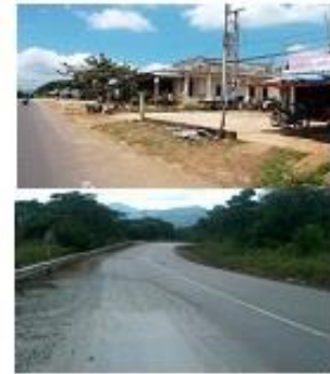
The NH19 before being rehabilitated.
