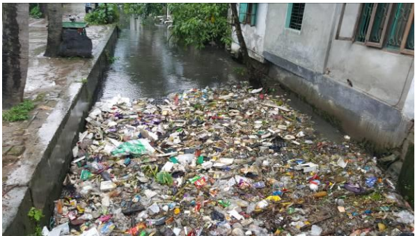
Dumping of solid waste into surface drain creating drainage congestion and environmental nuisance
