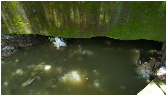
Figure 1: Existing drain at Cox’s Bazar pourashava
