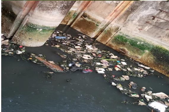
Drainage congestion due to disposal of solid waste in the drain
