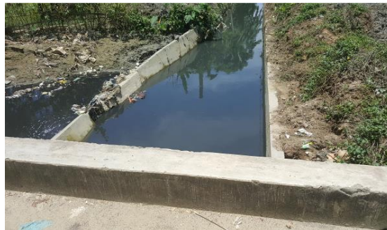
A drain with high turbidity and organic load of domestic sewage near Ocean Paradise hotel
