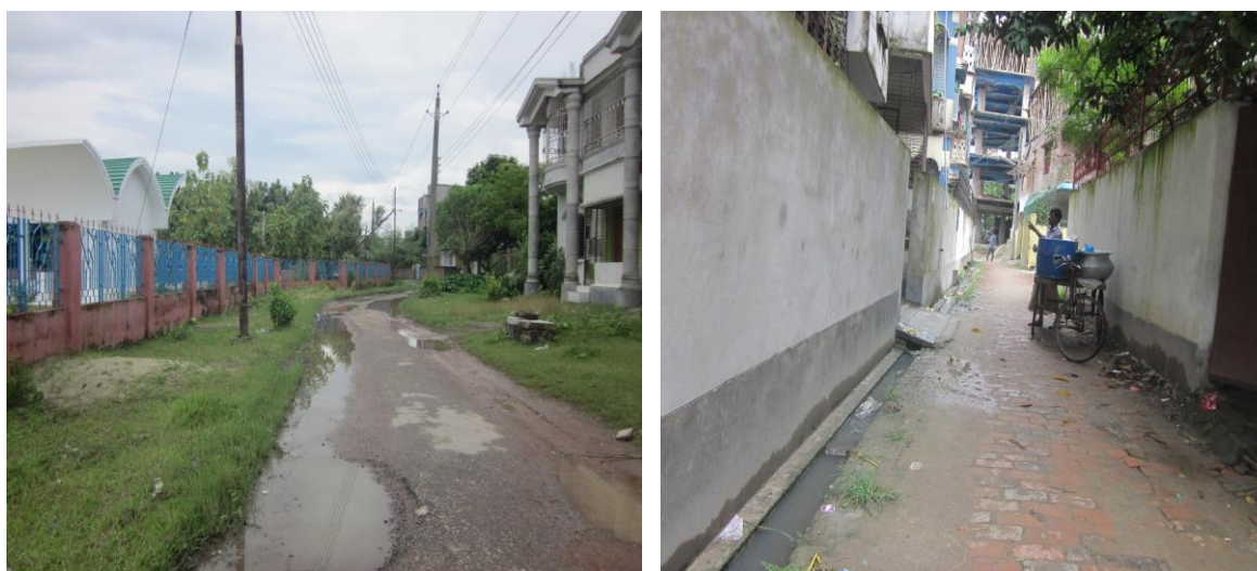
Figure 2: Existing damaged road and drain
