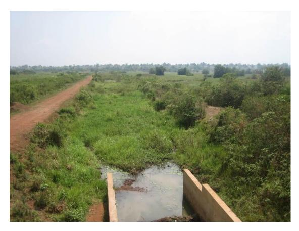
Figure 5: Silted/clogged canal in Itek-Kile rice scheme in Lira
