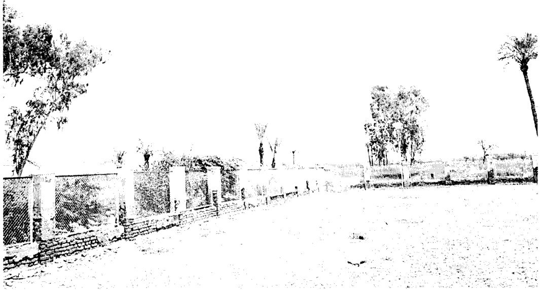
Photo 5: Place available for 132 Kv Grid Station in Existing boundary of 66 Kv Grid Station Choti
