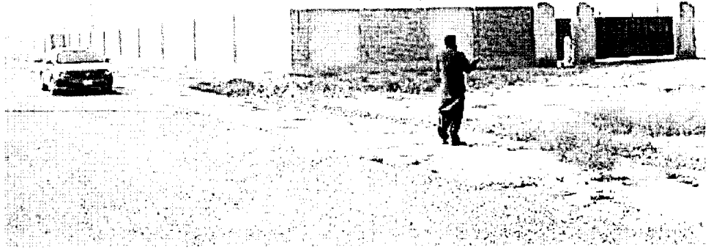
Photo 6: Site view of 132 KV New Grid Station Punjab Housing Society
