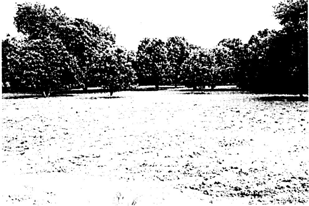
Photo 3: Site View of New 132 KV Buch Villas Grid Station
