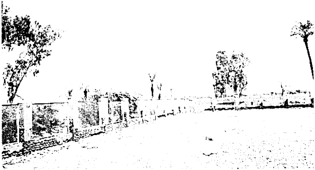
Photo 5: Place available for 132 Kv Grid Station in Existing boundary of 66 Kv Grid Station Choti
