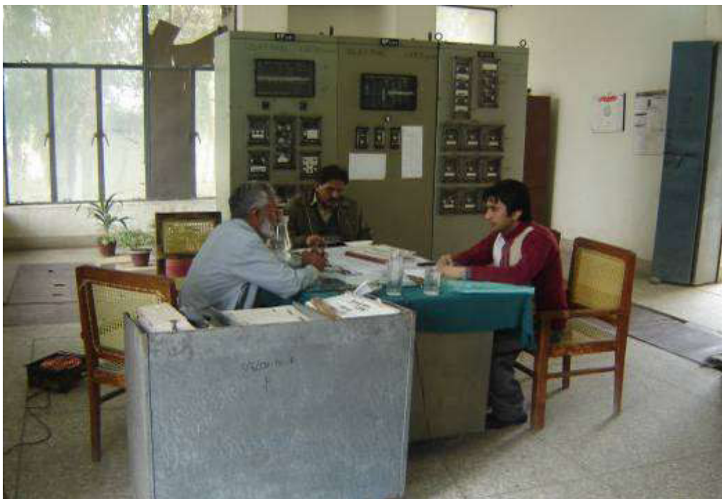
Public consultation at Lakarmar Grid Station with Station Officer (2009).
