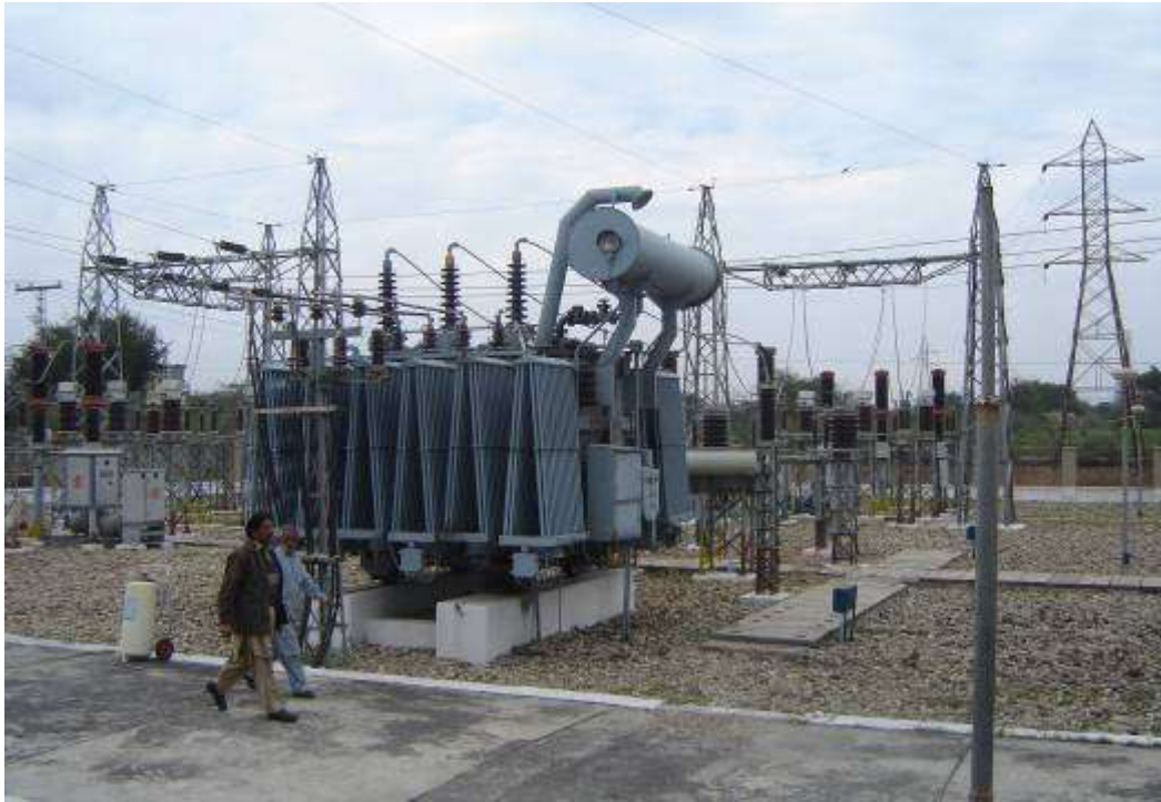
Showing existing status of 66KV Lakarmar Grid station yard and allied equipment.
