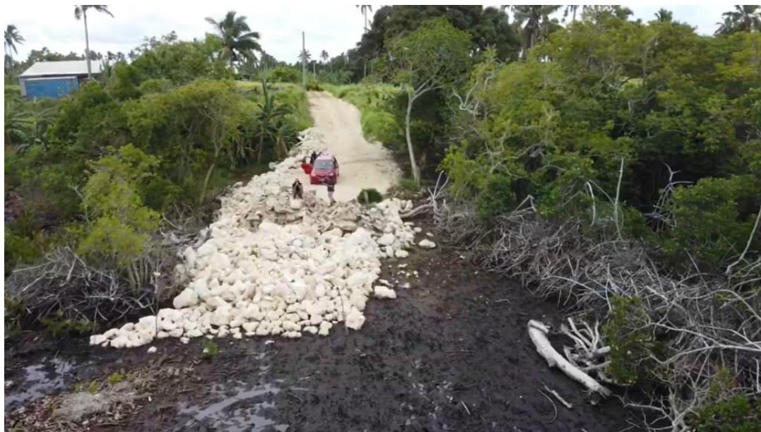
Plate 5.2: Reclamation and new access road through mangrove area
