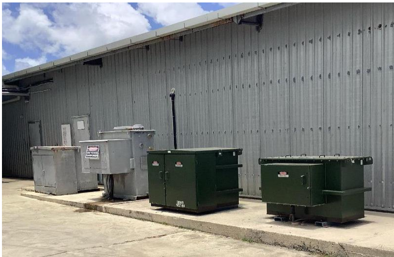
Ground-mounted transformers
