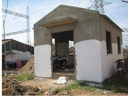
Hazardous waste storage area
