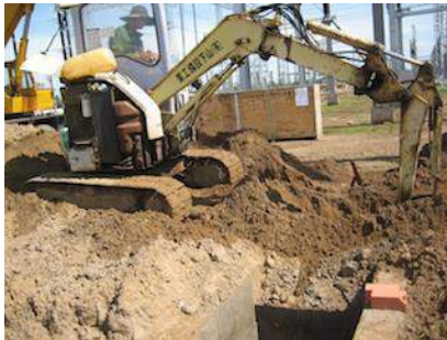
Surface grading activities causing soil runoff into the canal
