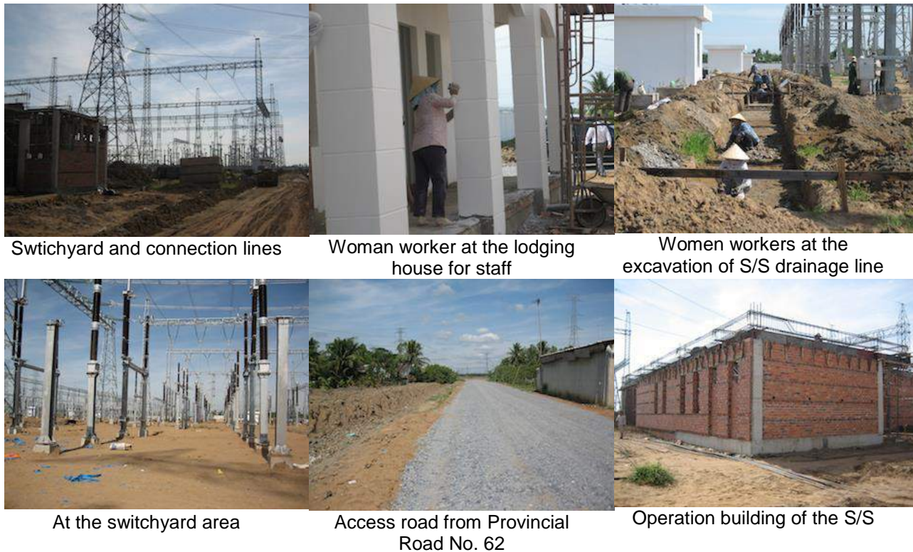
Photo 6: Ongoing construction activities at 500kV My Tho Substation
