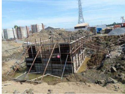
Oil containment tank
