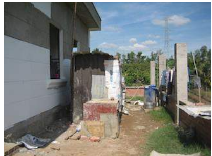
One of the common toilets
