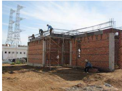
Workers without safety belt or harness
