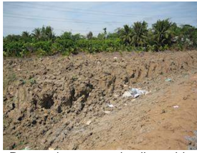
Dumped excavated soil outside the substation site
