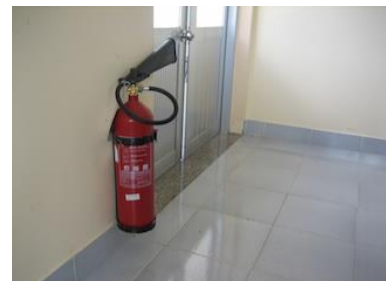
Fire extinguisher inside the operation building
