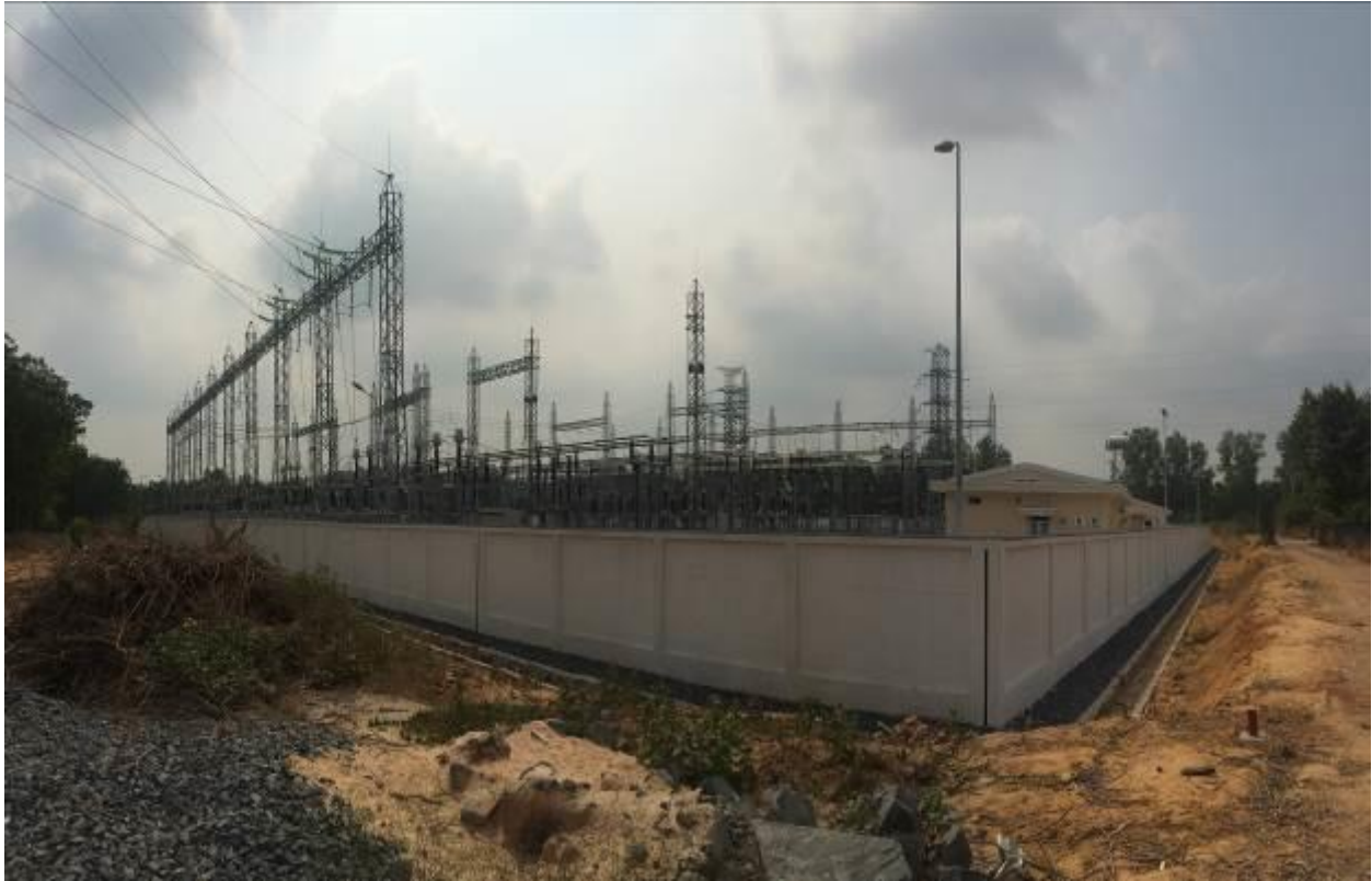
Surrounding of 220 KV Uyen Hung Substation
