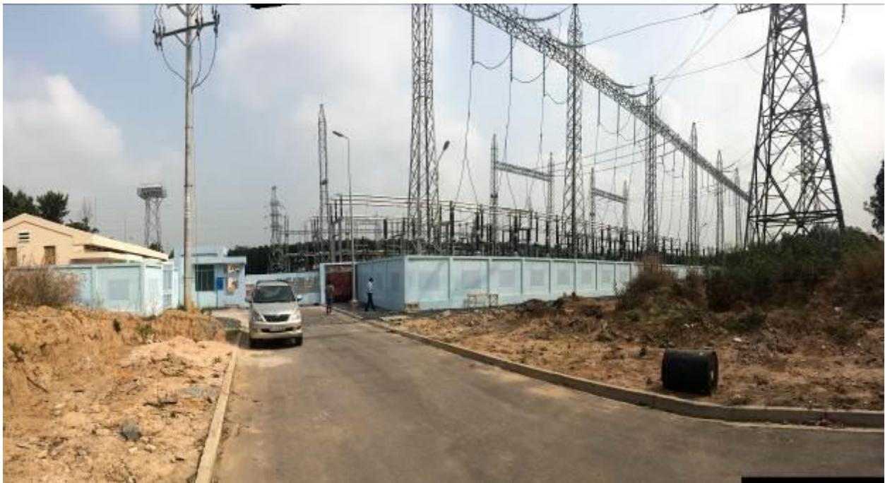
Site of the proposed access road
