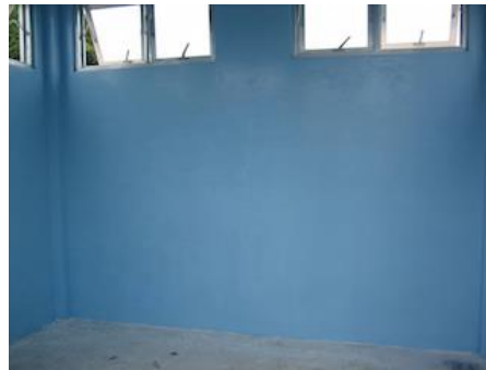
Inside the HW storage house
