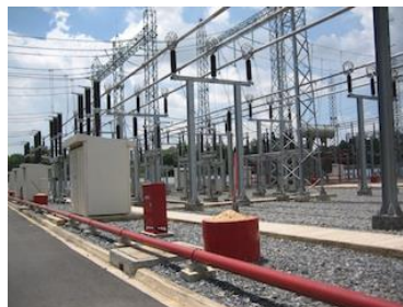
Fire suppressants at the SS
