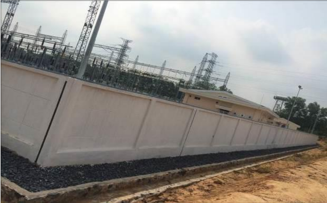
The drainage surrounding the substation
