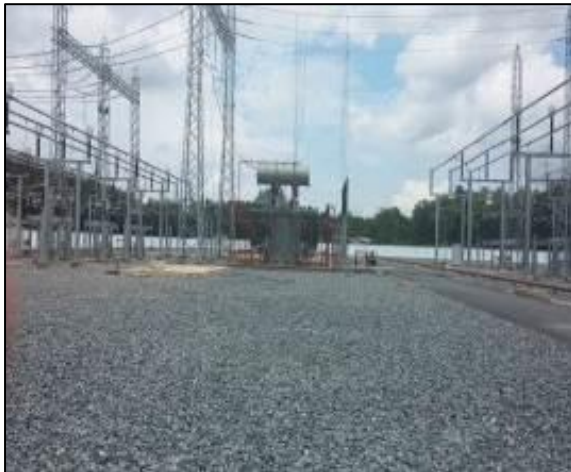
Current 250 MVA transformer
