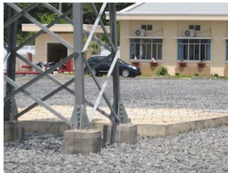
Photo 4: Oil Containment for Existing Transformer
