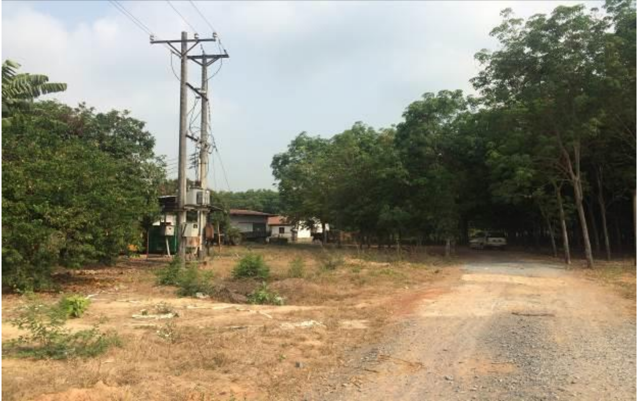
At the back of the substation is a house and the rubber tree plantation
