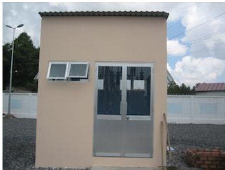
Hazardous waste storage house
