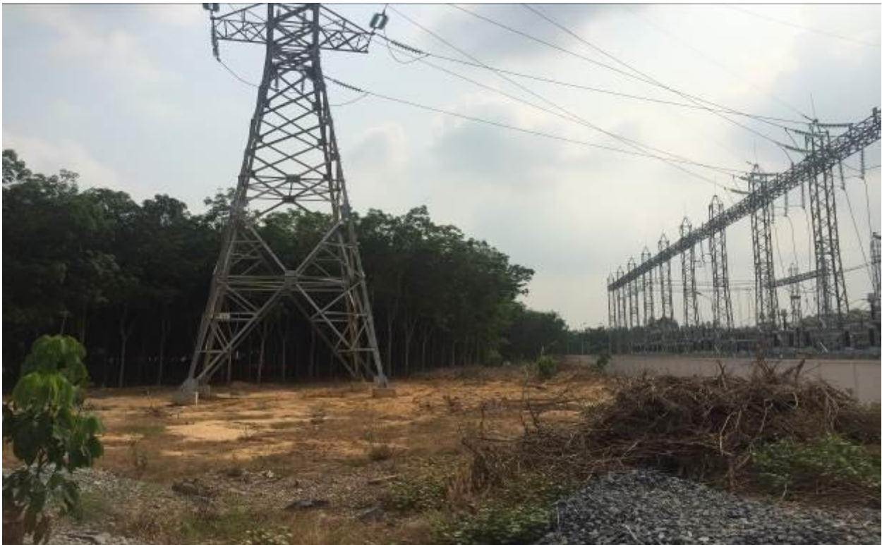
Rubber tree plantation adjacent to the substation
