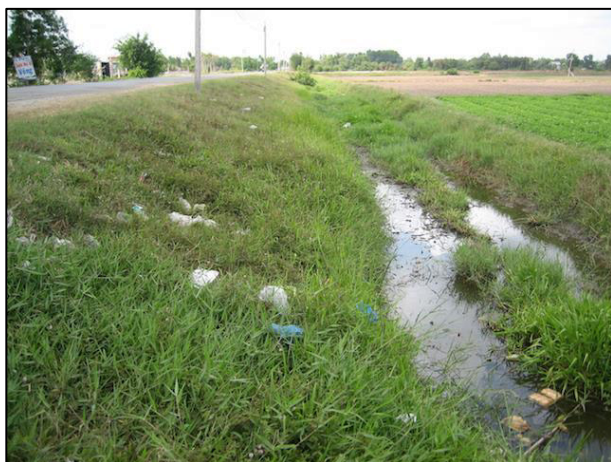
Irrigation canal at western area of S/S
