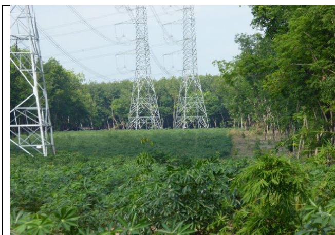
Fig 4a: Substation will be located in rubber plantation area right of dual towers.
