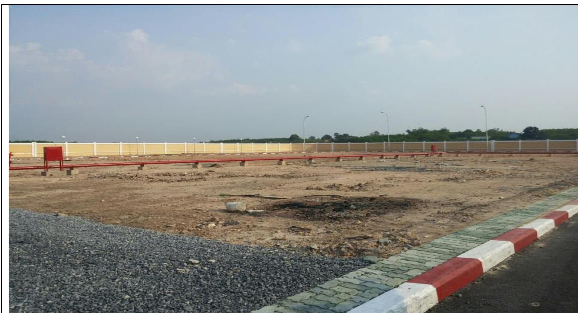
Fig 5c: Location inside substation for 2 nd substation
