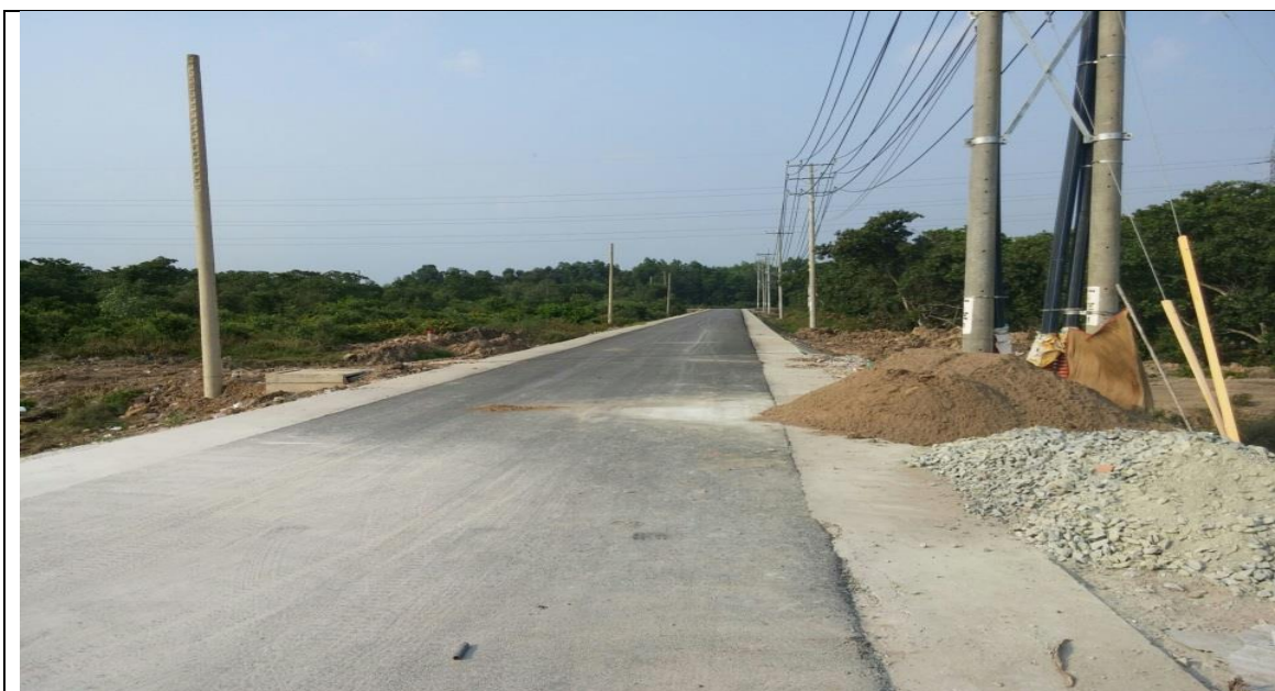
Fig 5a: Access road to the substation
