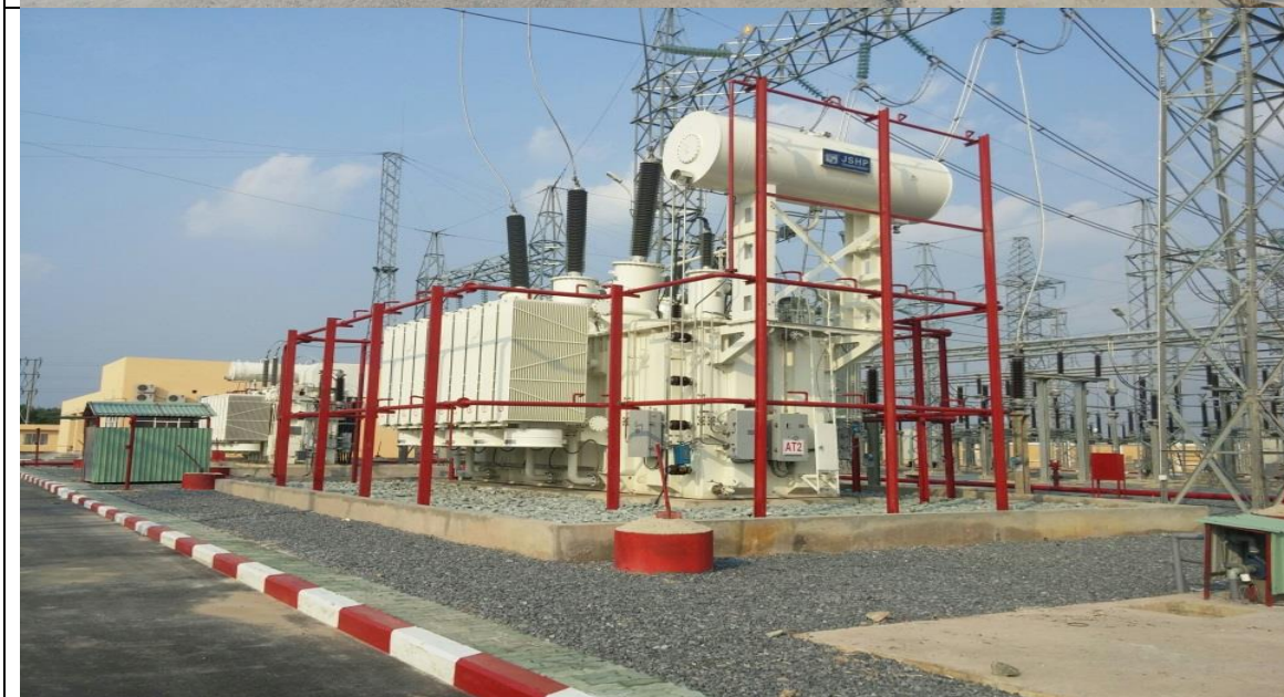
Fig 5b: The 1 st transformer installed
