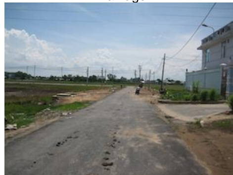
Access road to substation next to staffhouse
