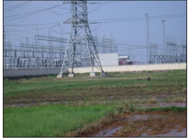
Riceland at the eastern area of the substation
