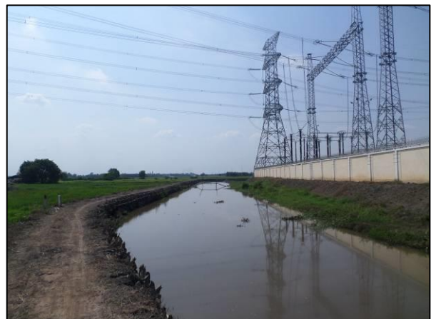
Irrigation canal at southern area of S/S
