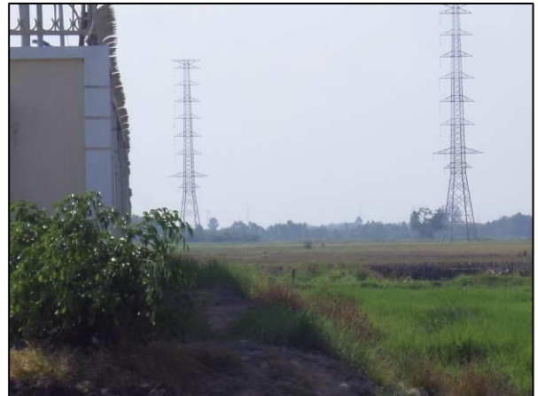
At the northern section of the substation
