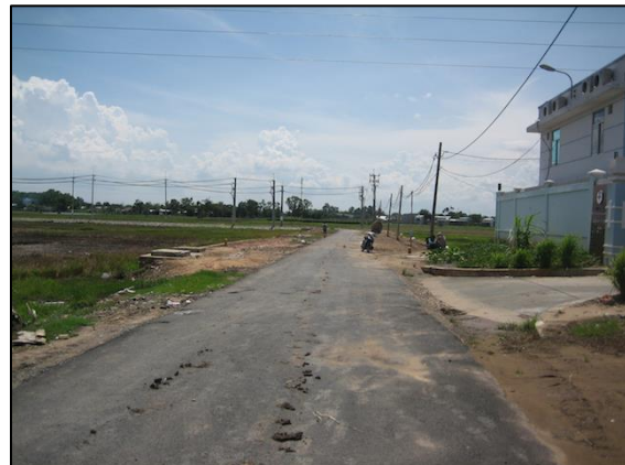
Access road to substation
