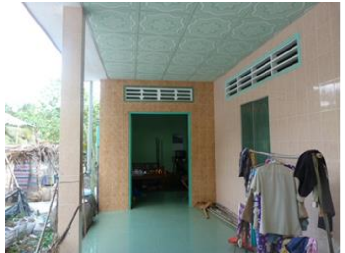
The affected house area
