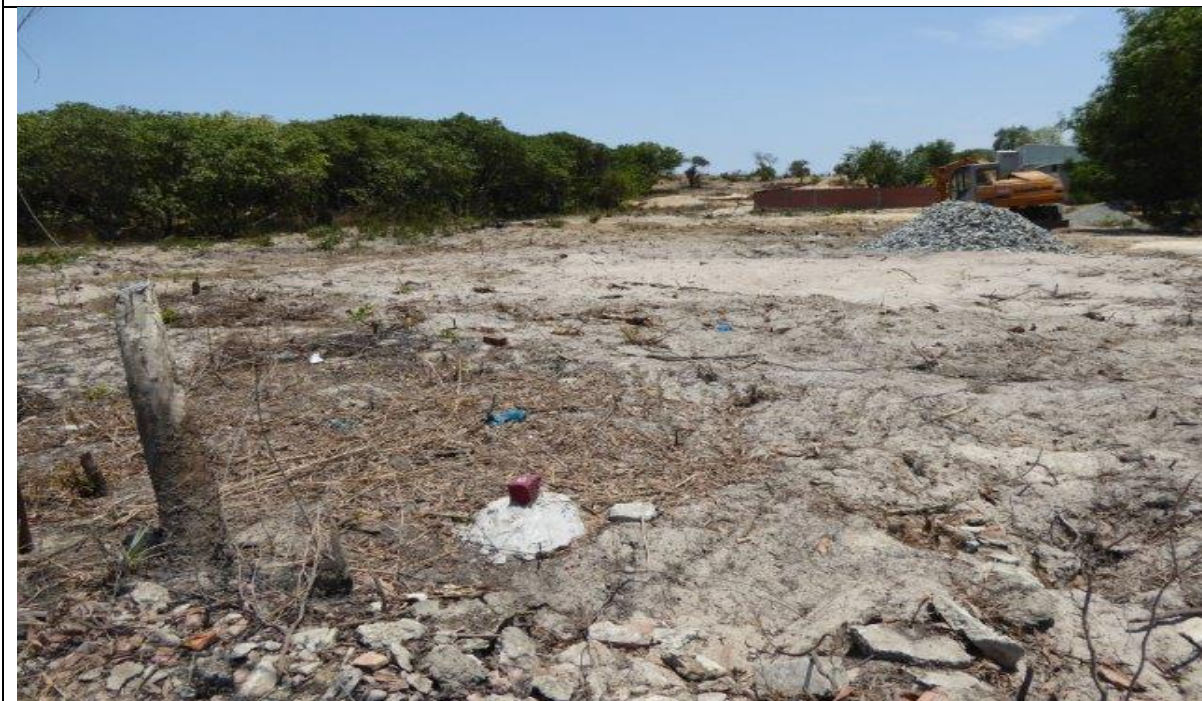
Fig.5b: ROW for new access road to substation
