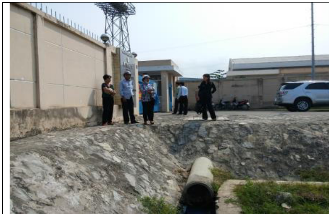
Fig 4a: Gate of substation
