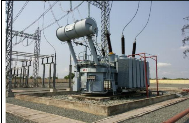
Fig 4b: Existing Transformer
