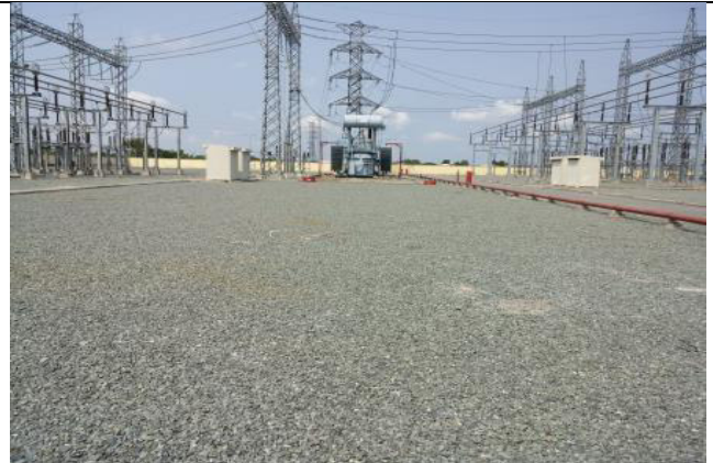
Fig 4c: Location for new transformer
