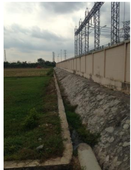
Drain system around the 220/110 kV Tra Vinh Substation
