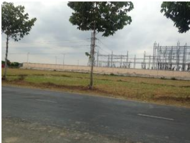
Outside the 220/110 kV Tra Vinh Substation
