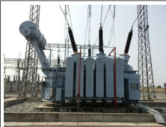
Transformer 1 in the existing 220/110 kV Tra Vinh substation
