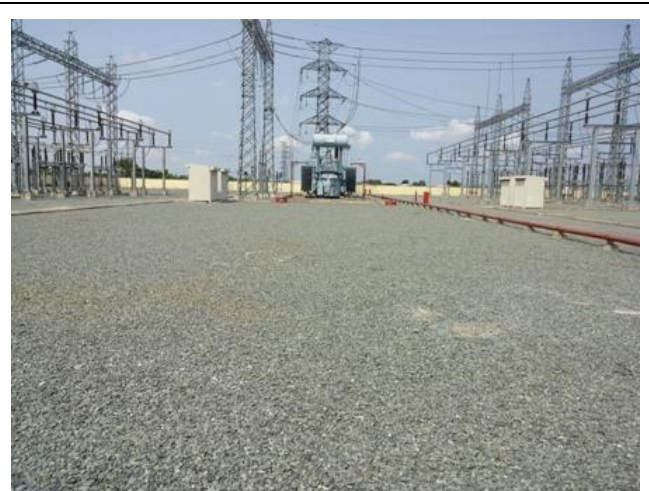
Inside existing 220/110 kV Tra Vinh substation
